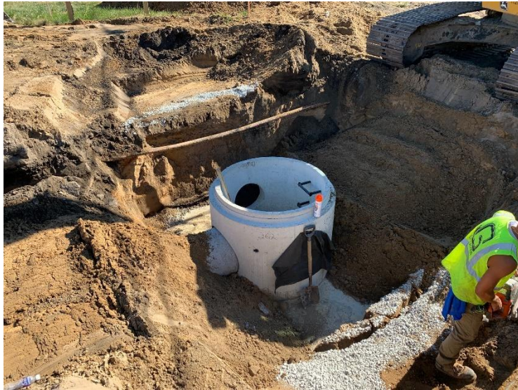
Figure 1: Grimmer Installs Manhole
