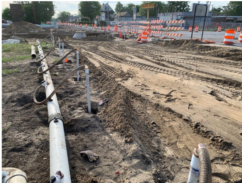
Figure 2: Jobsite looking East towards Future Roundabout
