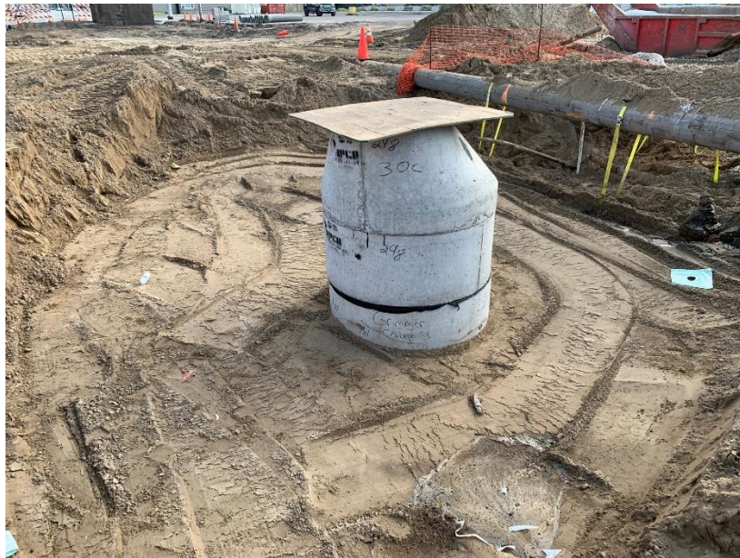
Figure 1: Grimmer Installed STR 248 M-Type Manhole
