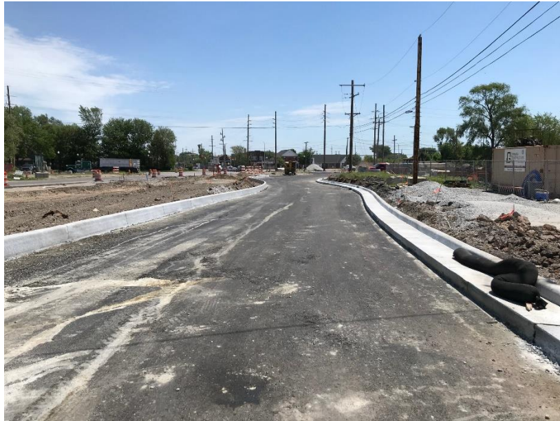
Figure 2: Curb and Gutter Looking East on Gostlin
