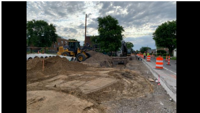
Figure 2: Jobsite looking East from Future Roundabout
