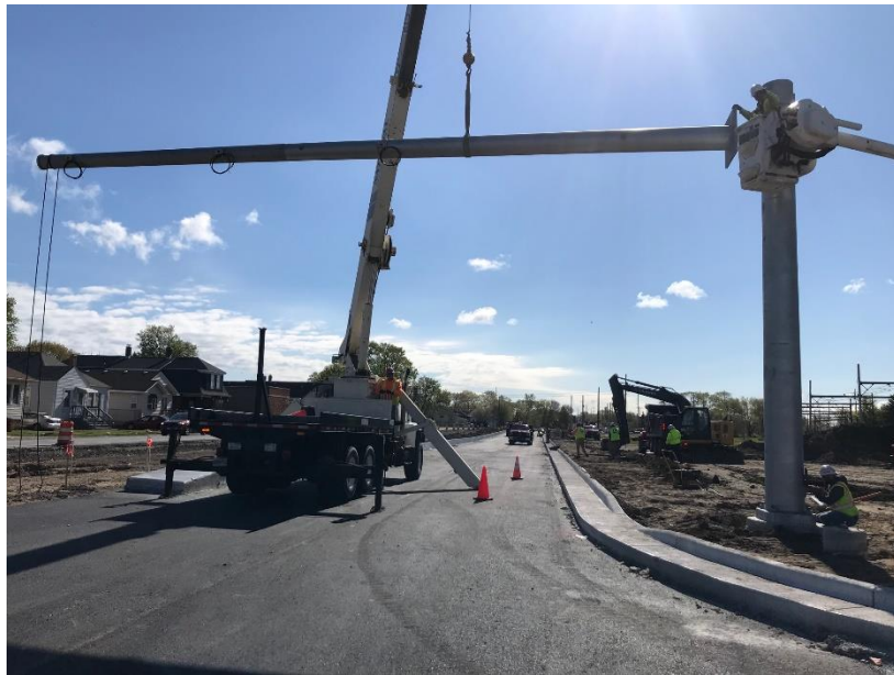
Figure 1: Hawk Erects Mast Arm at Dearborn
