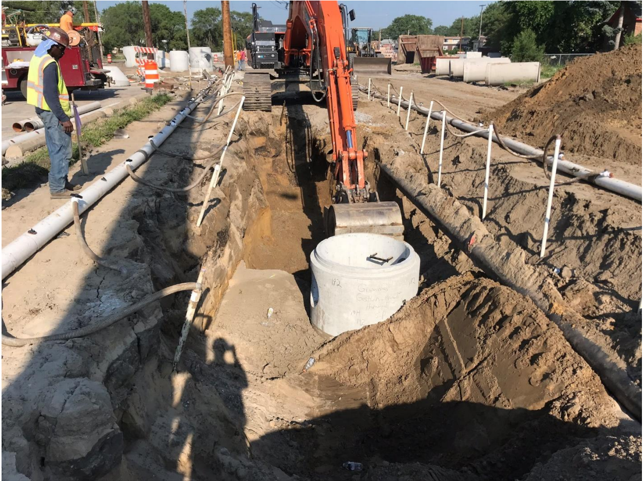
Storm installation with manhole
