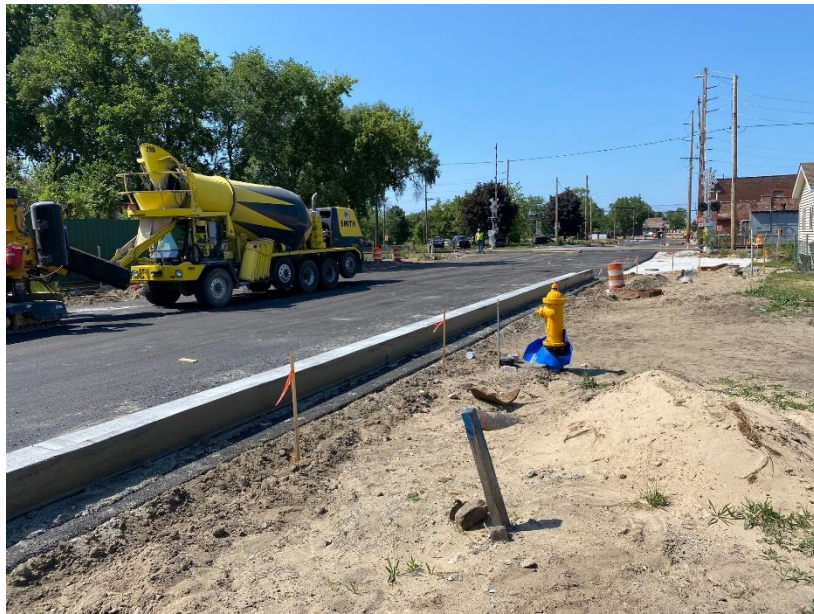
Figure 2: Milestone slip forms curb and gutter
