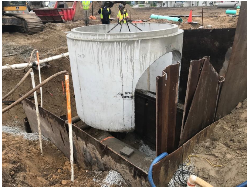
Figure 1: Grimmer Installs STR 248 M-Type Manhole
