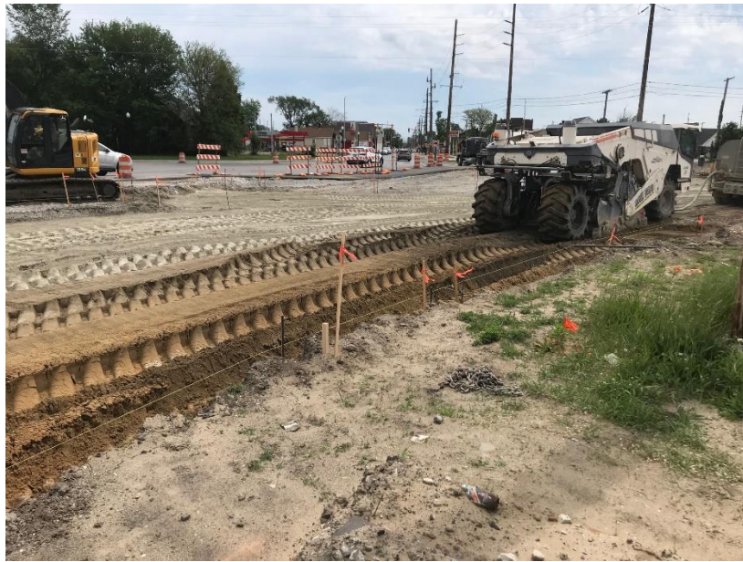
Figure 1: Rock Solid Chemically Modifies Subgrade
