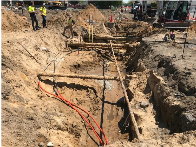
Figure 1: CenturyLink Creates Space for Grimmer to Install M-Type Manhole
