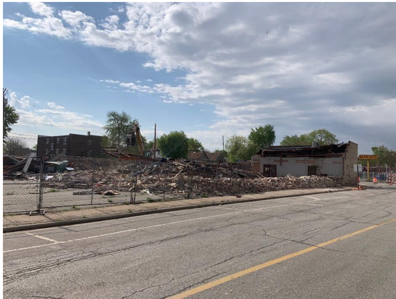
Figure 1: JM Wrecking Demoing Ace Hardware
