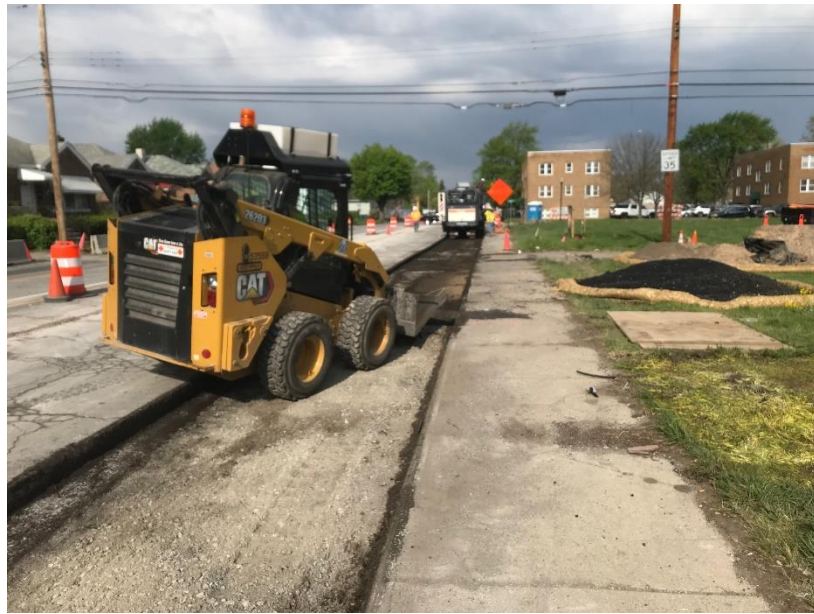
Figure 2: Milestone Mills out HMA Pavement
