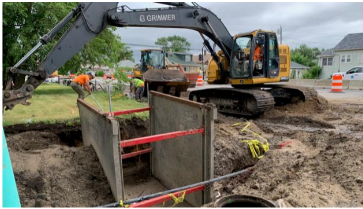
Figure 1: Grimmer works at Cameron
