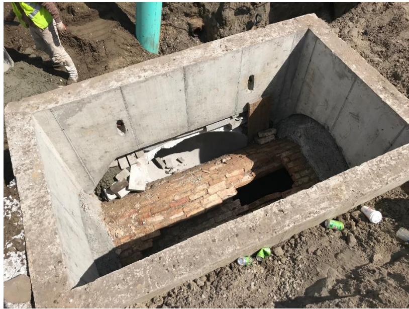
Figure 2: New Structure over Existing Brick Sewer
