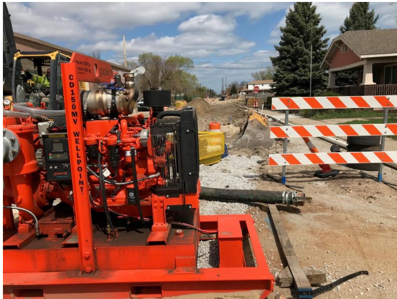
Figure 1: Dewatering Pump on Sheffield
